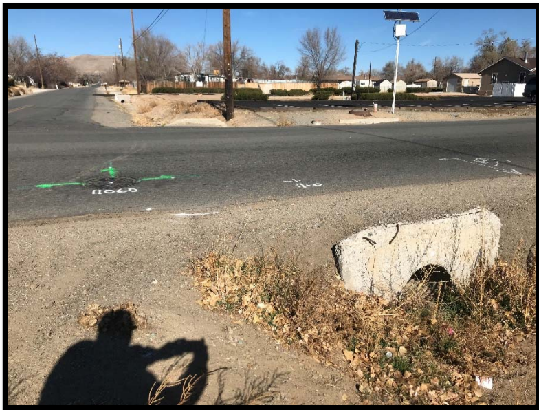
Figure 8 – Culvert crossing E. 4 th Avenue
